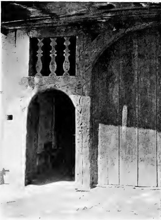
490 ENTRANCE TO A HOUSE AT WOJKOWICE
